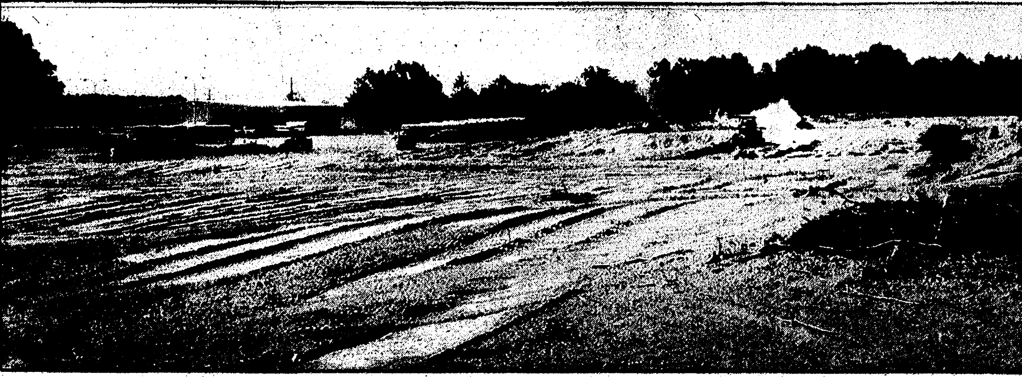
—New Elementary in Progress—
